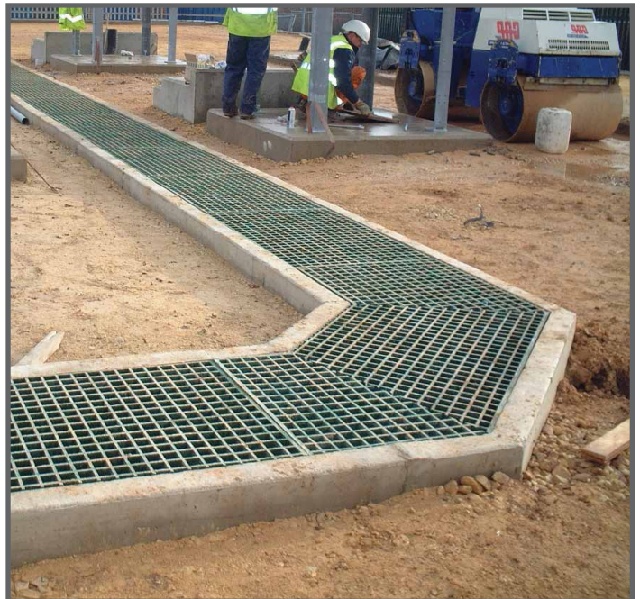
After Installation of FRP Trench Covers
