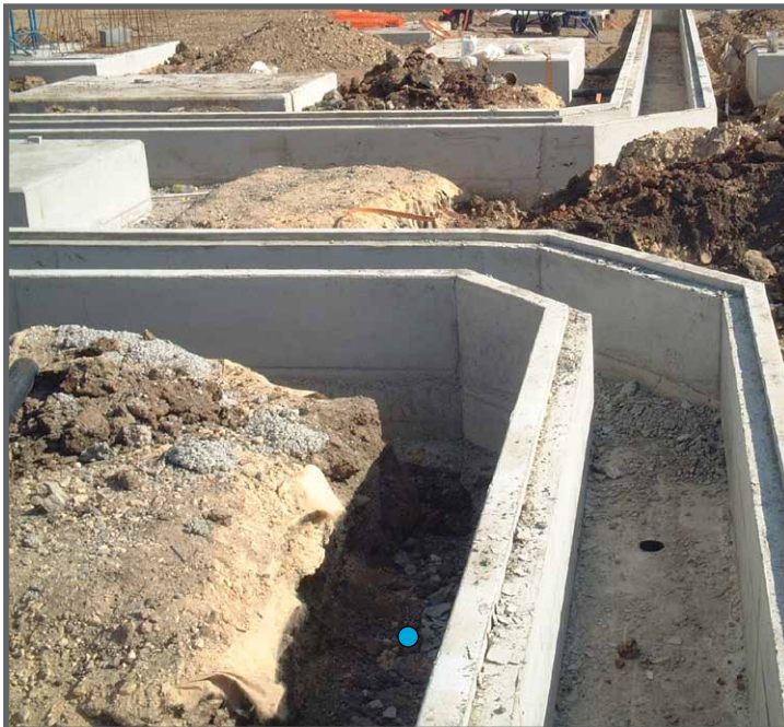
During Construction of Utility Trench
