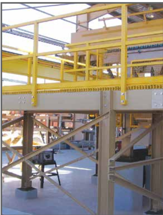
Fibergrate structural shapes and pultruded grating were used in this mining facility for their corrosion resistance.
