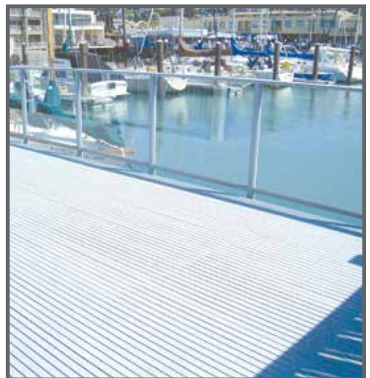
Fibergrate® FRP products replaced rotting wood at this yacht club. The new surface is corrosion and slip resistant plus barefoot friendly.
