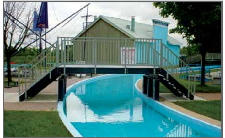
This bridge at a waterpark was constructed using Fibergate's railings, grating, stair treads and structural shapes. In addition to being ADA compliant and slip resistant, this grit-top surface is also barefoot friendly.
