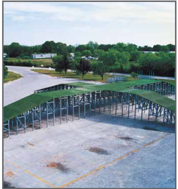
This all FRP (fiberglass reinforced plastic) structure was specifically designed for a General Dynamics anechoic testing chamber. FRP was required because its properties are transparent to the radio and electromagnetic waves used during aircraft testing.
