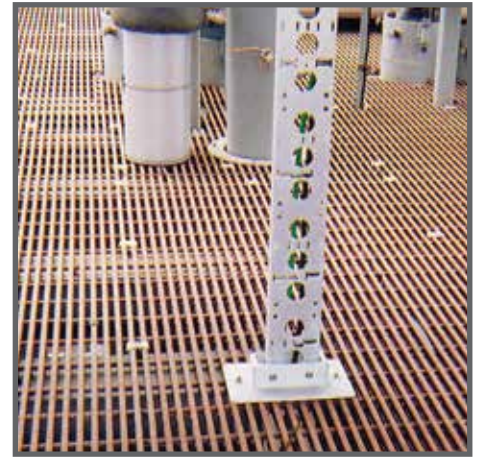
Offshore Oil & Gas Platform
