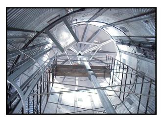
Fibergrate's Dynaform® structural shapes were used in constructing the frame, while Fiberplate® (fiberglass reinforced plastic plate) was used to create the dome's exterior. Not only did Fibergrate create an aesthetic structure, the FRP components won't interfere with the antenna signals.
