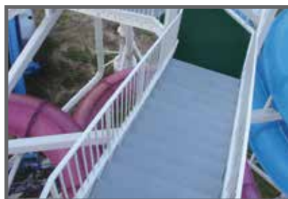
Covered stair treads, with hidden hold down clips, lead to a water slide at a municipal waterpark in Oklahoma.
