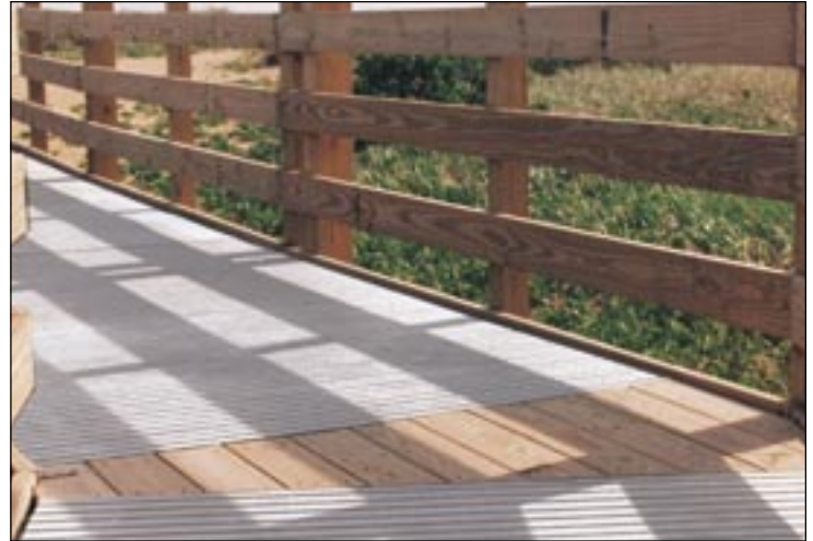
Safe-T-Span pultruded pedestrian grating was chosen by EAN Corporation for this walkway bridge for swimmers at South Cape Beach State Park near the Cape Cod region of Massachusetts.
