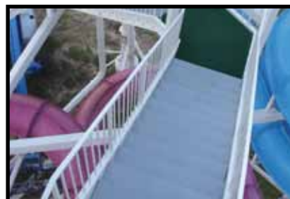
Covered stair treads, with hidden hold down clips, lead to a water slide at a municipal waterpark in Oklahoma.
