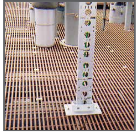
Offshore Oil & Gas Platform
